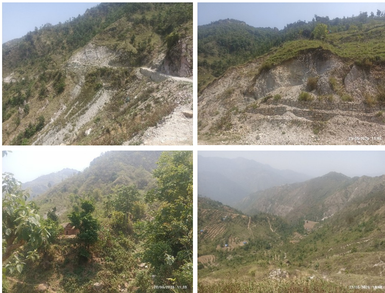
Photograph 76 Landslide Site, Dapcha
