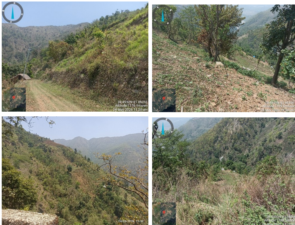
Photograph 90 Landslide Site, Kapase
