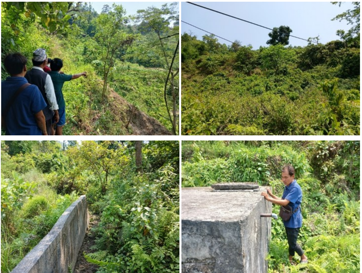
Photograph 39 Landslide Site, Purbe Kharpani
