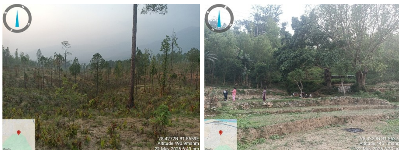
Photograph 74 Landslide Site, Gangate Khola
