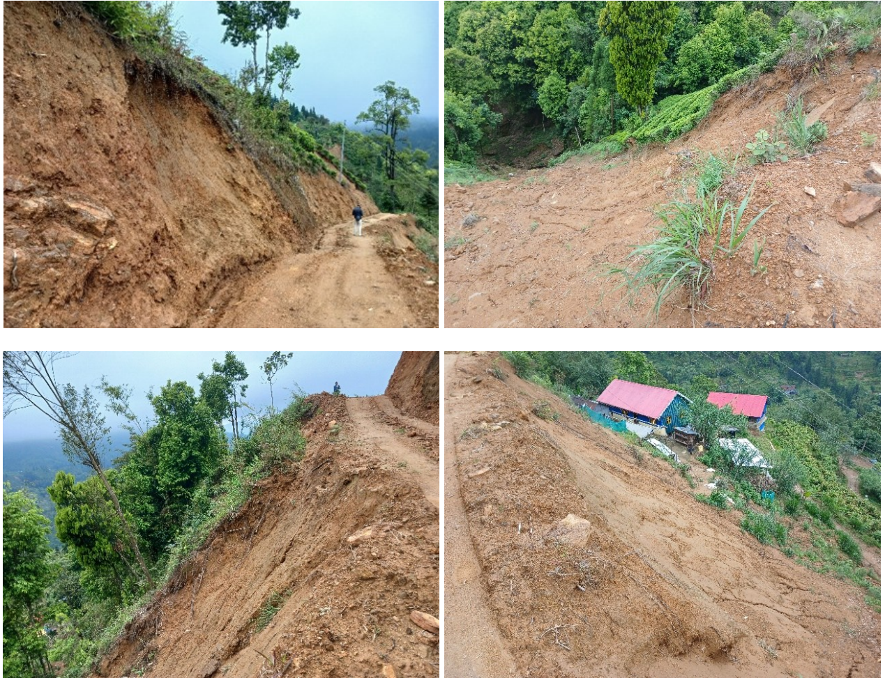
Photograph 10 Landslide Site, Manedanda Tol
