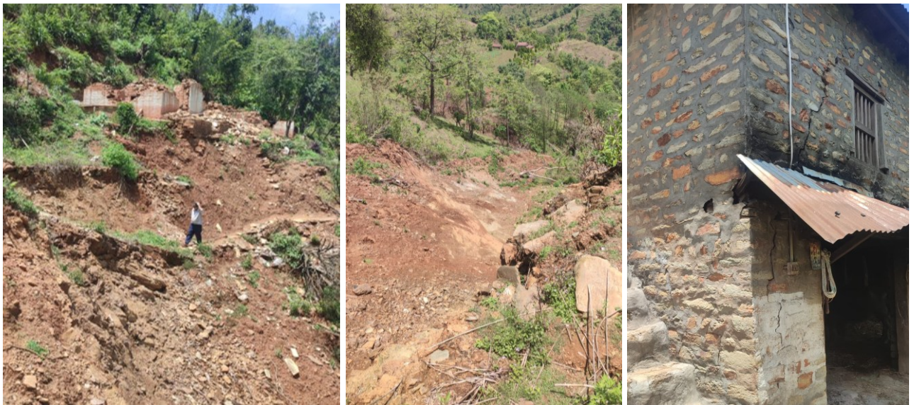
Photograph 58 Landslide Site, Kbalte
