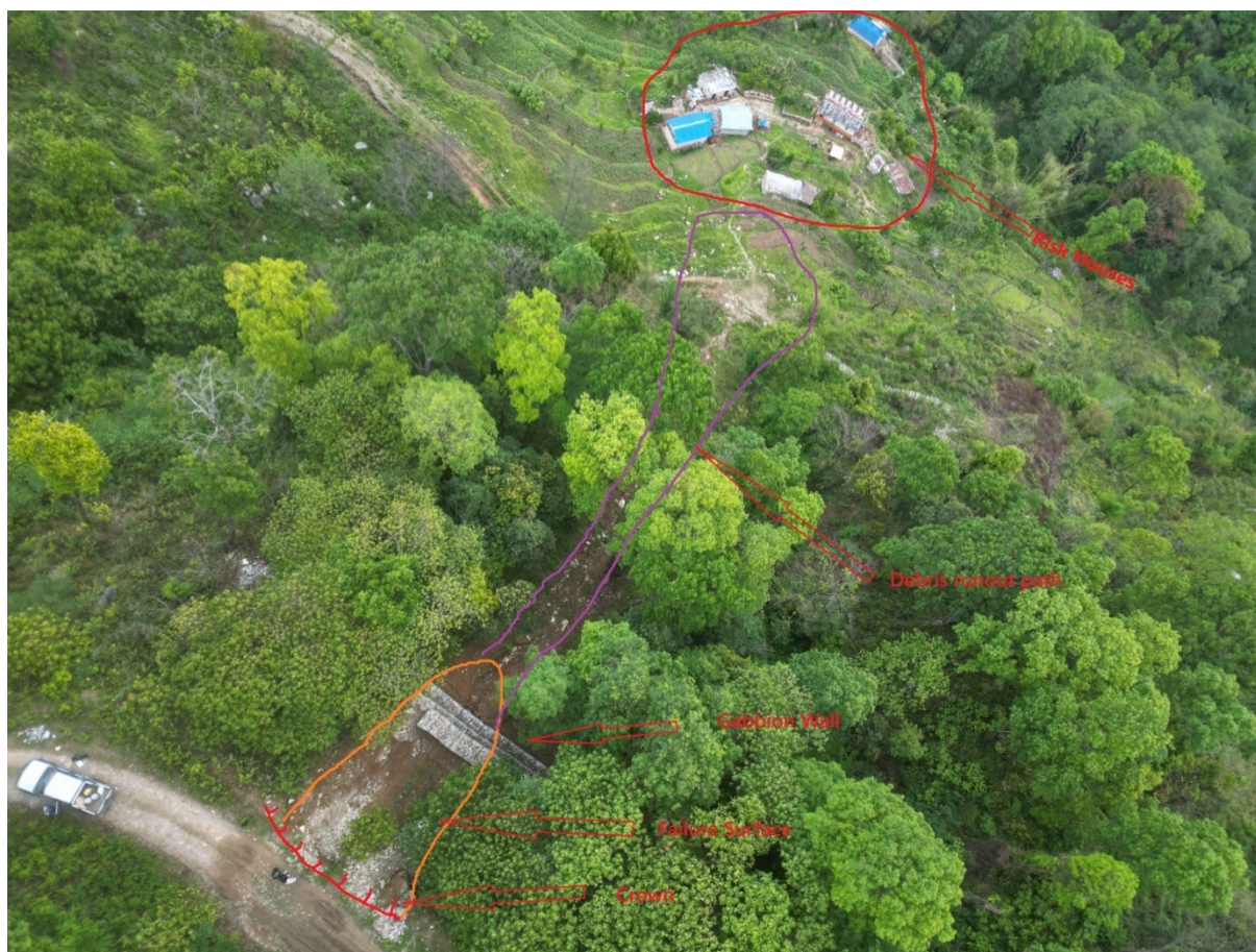
Photograph 59 Landslide Site, Okhrani Kalamuda
