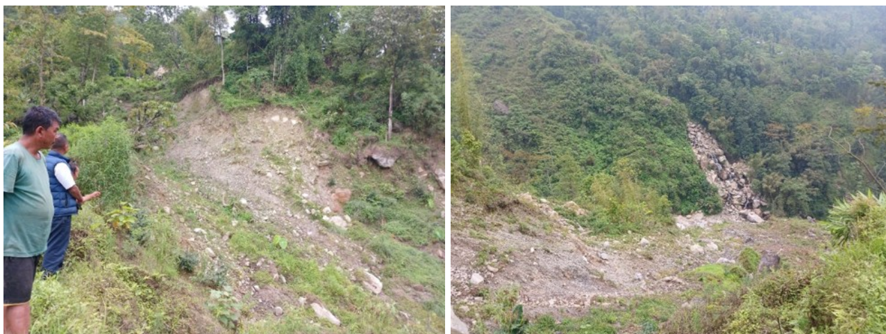
Photograph 22 Landslide Site, Ambe Tol
