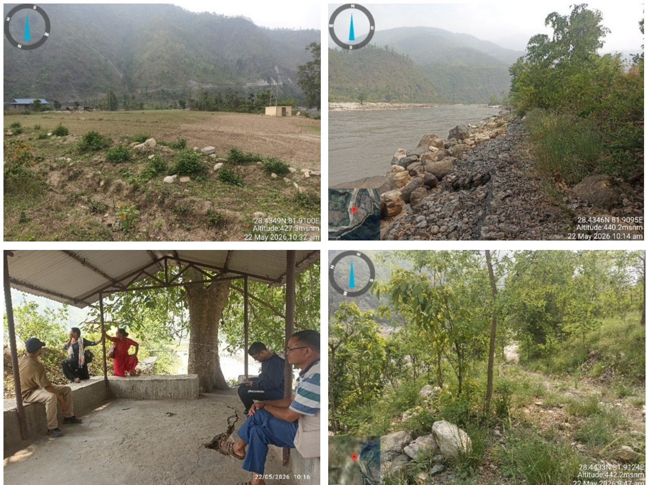
Photograph 78 Landslide Site, Bhulke
