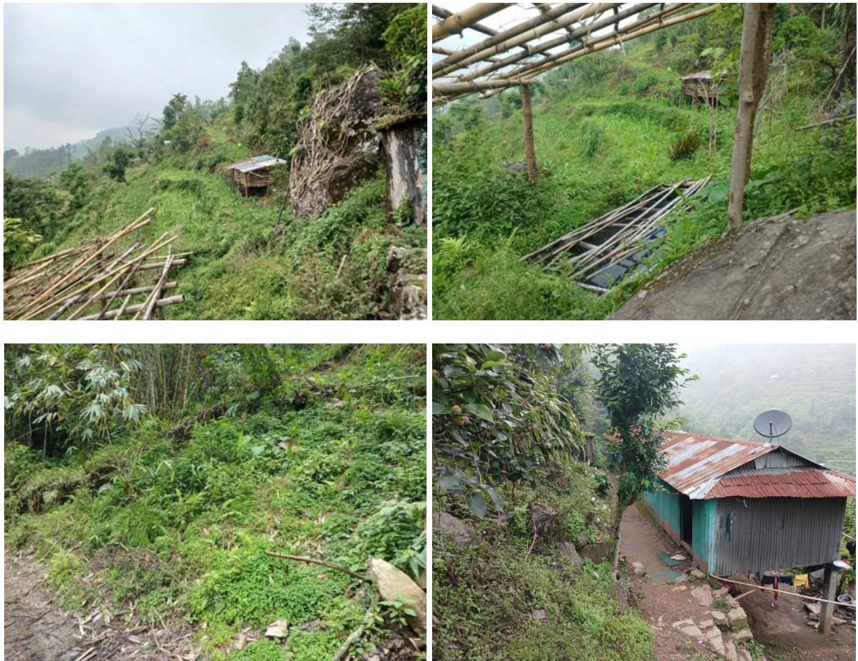
Photograph 31 Landslide Site, Sundarbasti Tol
