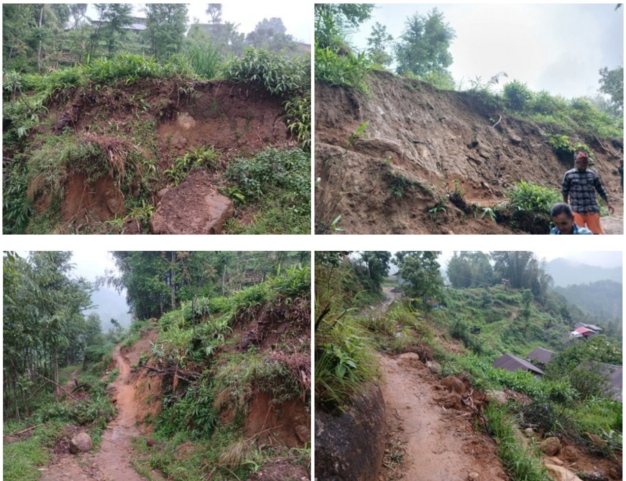
Photograph 4 Landslide Site, Ghising Gaun (Makarjung)
