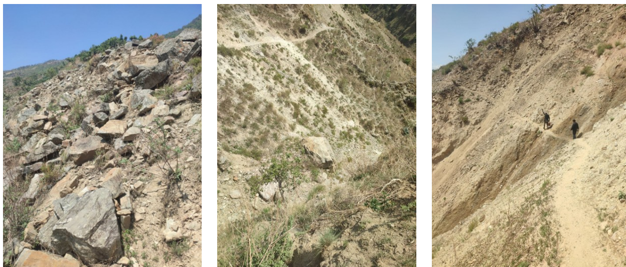
Photograph 94 Landslide Site, Thulo Madu, Bade, Buase
