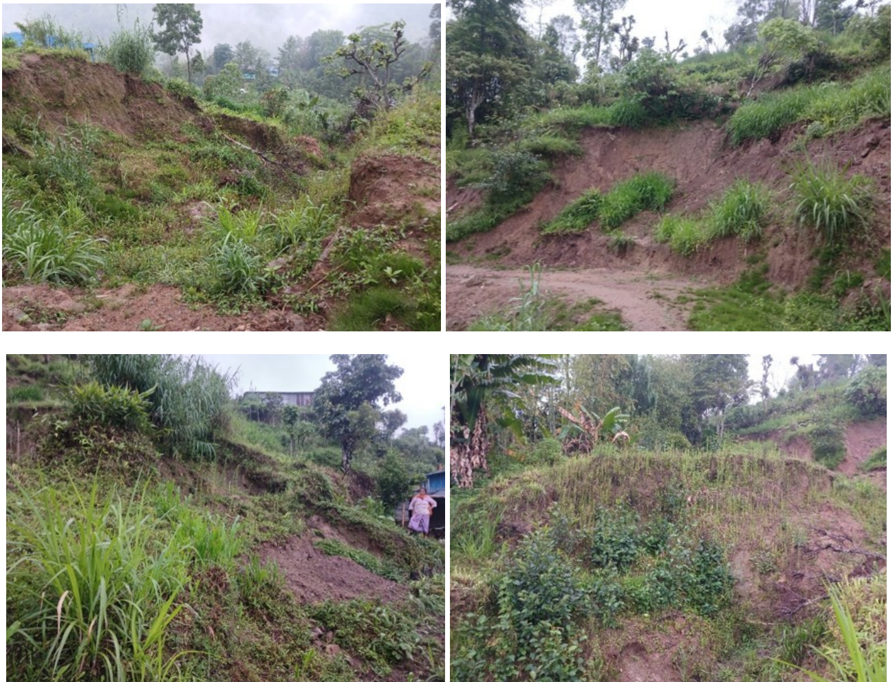
Photograph 15 Landslide Site, Mehelbote
