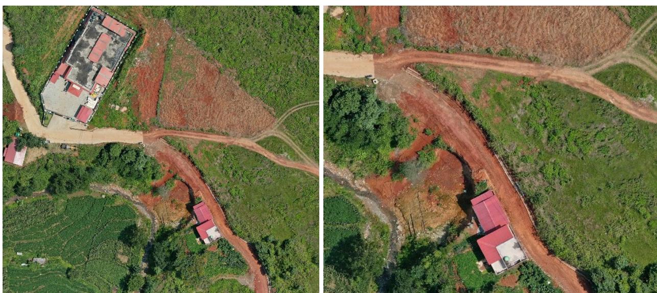
Photograph 56 Landslide Site, Nagarpalika Office
