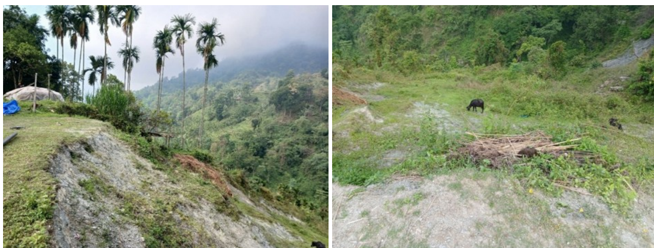
Photograph 38 Landslide Site, Sabakale Tol
