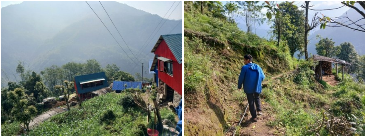
Photograph 44 Landslide Site, Todke
