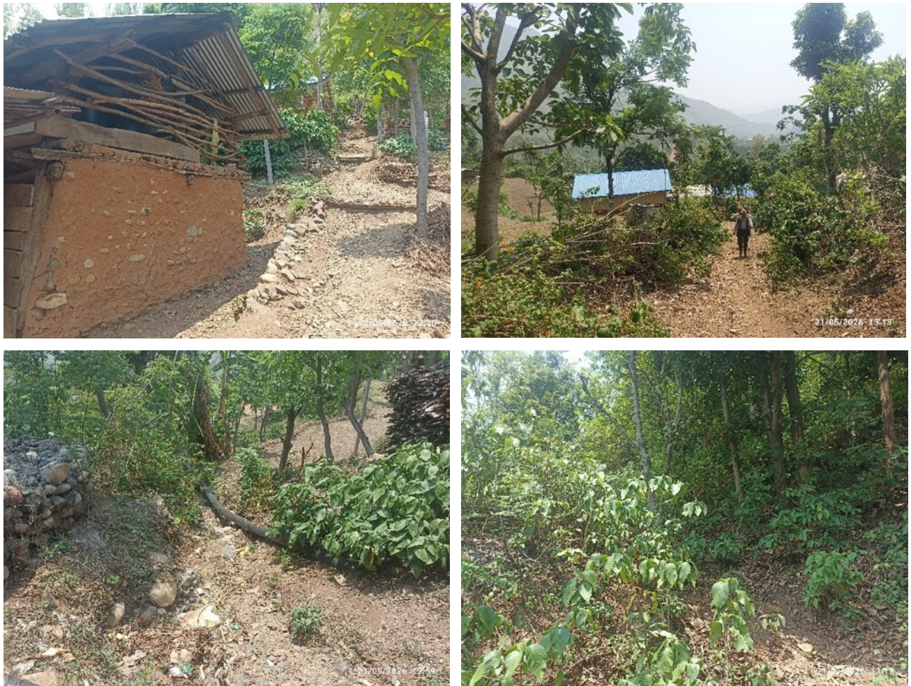
Photograph 82 Landslide Site, Barmagar
