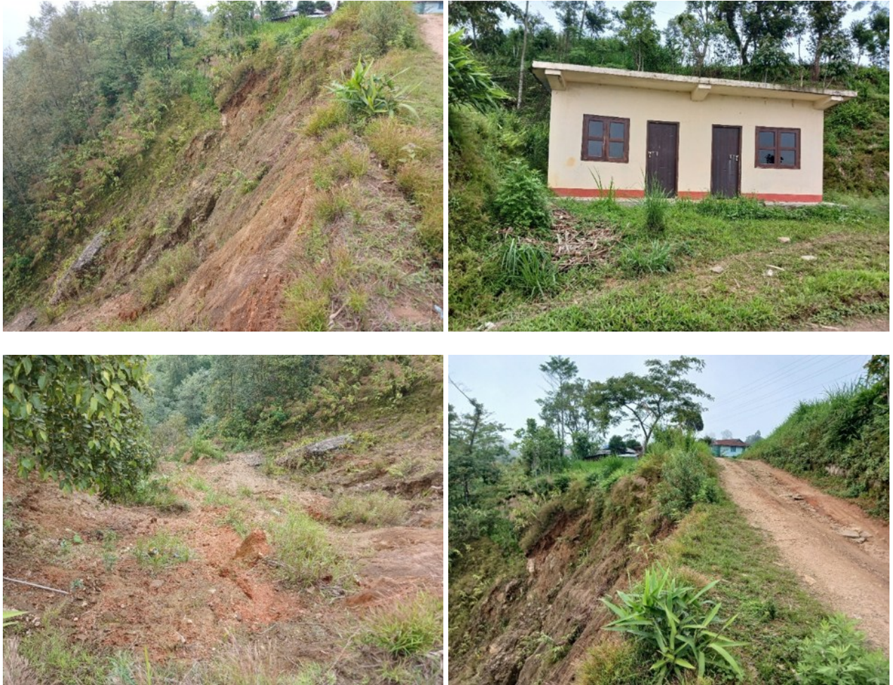
Photograph 36 Landslide Site, Thulo Bardu Tol
