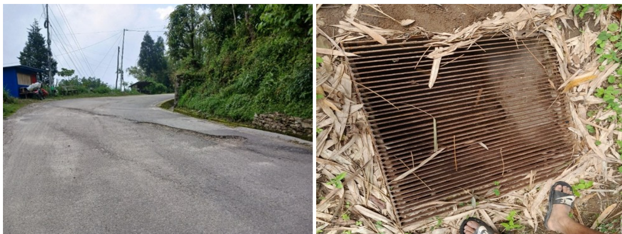
Photograph 27 Landslide Site, Bhalu Khop
