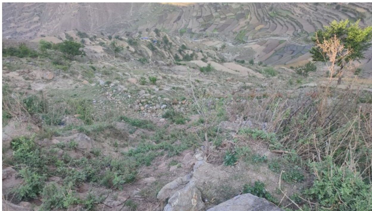
Photograph 93 Landslide Site, Jogkbhola, Dalit Basti
