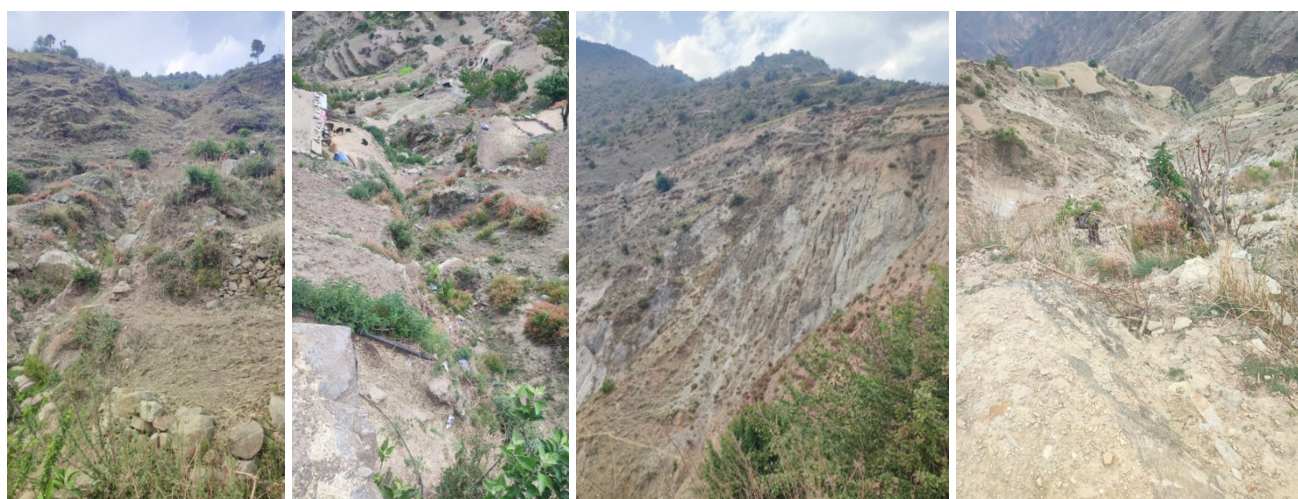
Photograph 91 Landslide Site, Kam Basti
