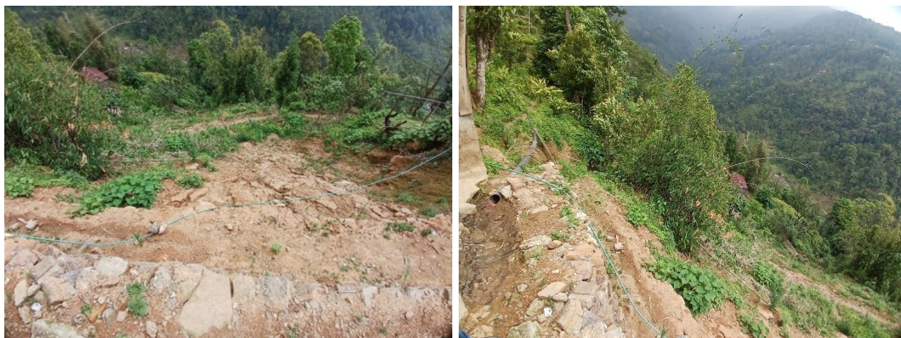
Photograph 7 Landslide Site, Khadka Gaun (Indreni Tol)
