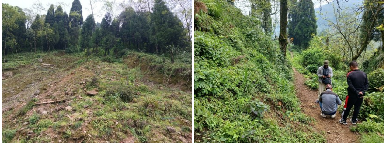
Photograph 8 Landslide Site, Manebhanjyang (Sunakhari Tol)
