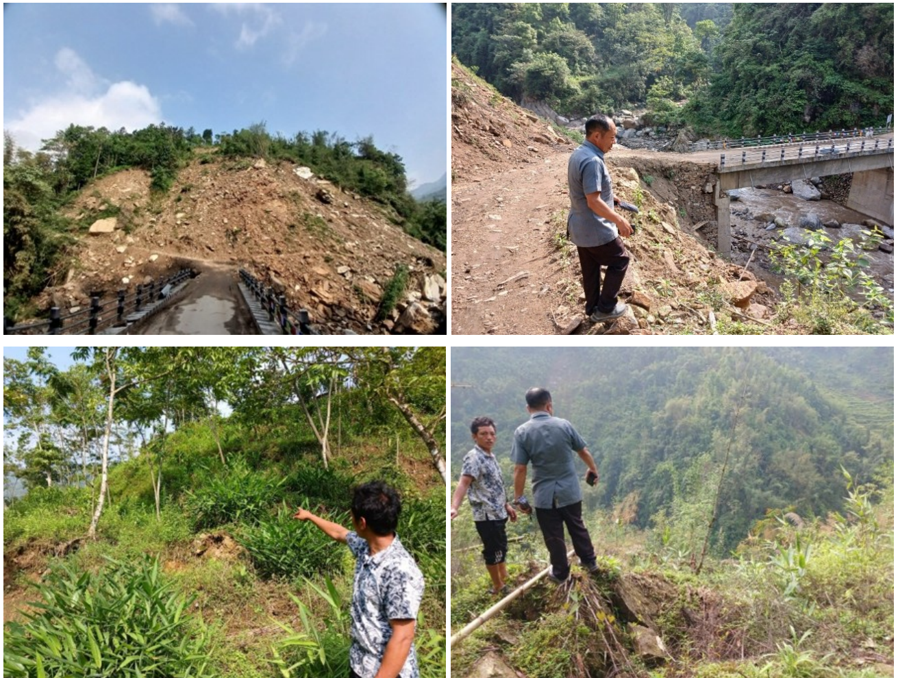
Photograph 46 Landslide Site, Gairigaun
