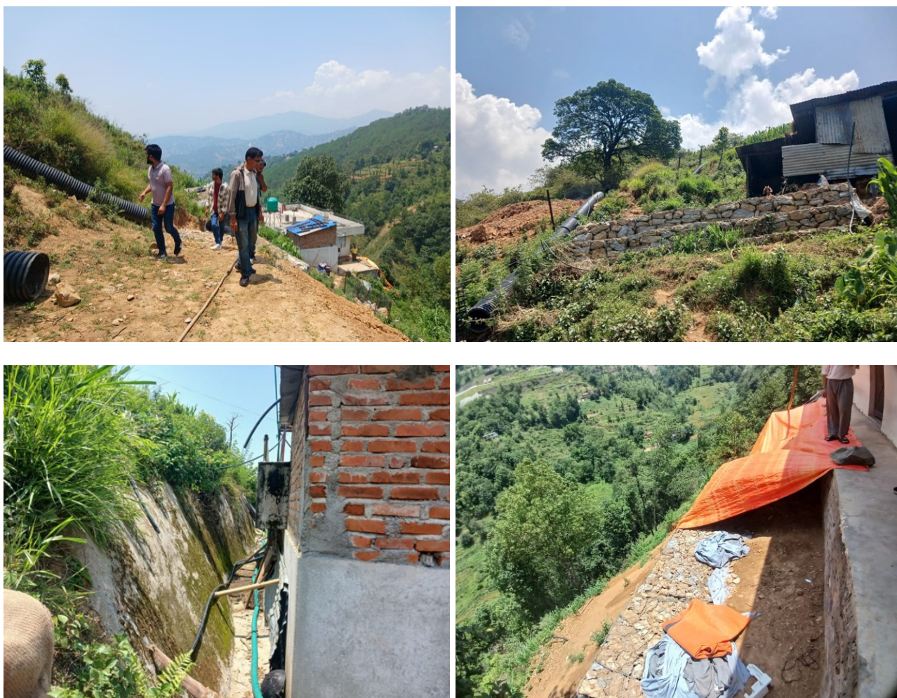
Photograph 55 Landslide Site, Khatri Pounva
