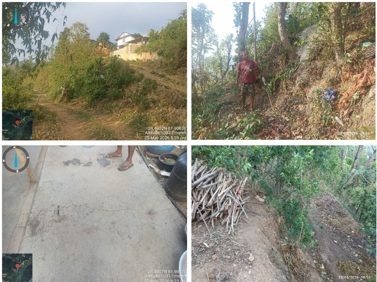
Photograph 75 Landslide Site, Nadekkot
