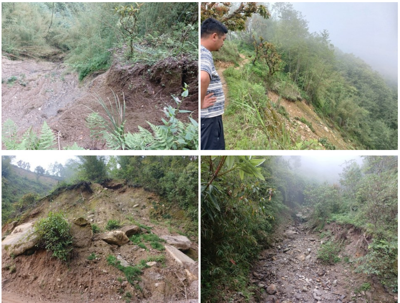
Photograph 45 Landslide Site, Kamere
