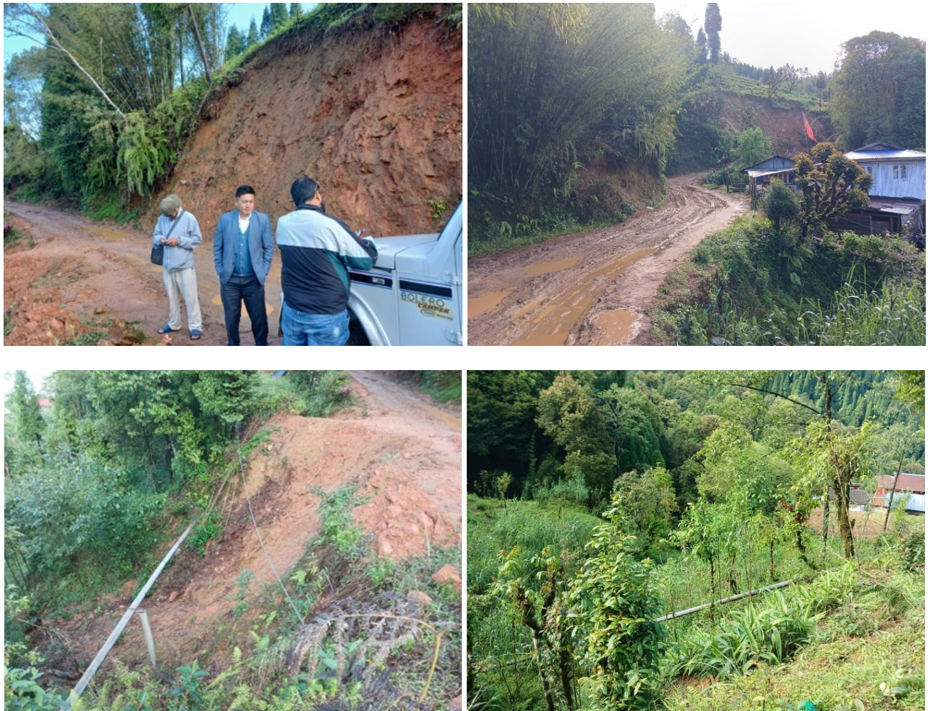
Photograph 14 Landslide Site, Makhamali Tol
