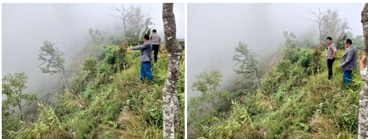
Photograph 30 Landslide Site, Deurali Tol
