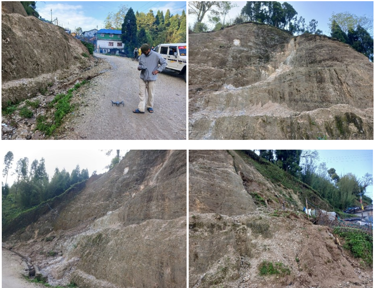
Photograph 12 Landslide Site, Deurali Tol
