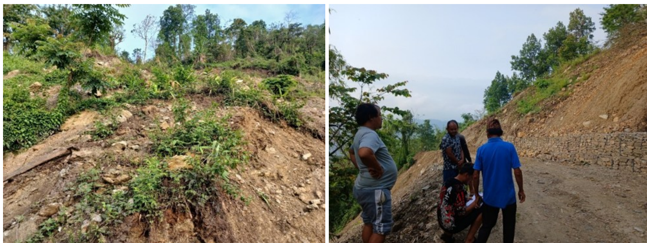
Photograph 37 Landslide Site, Simle
