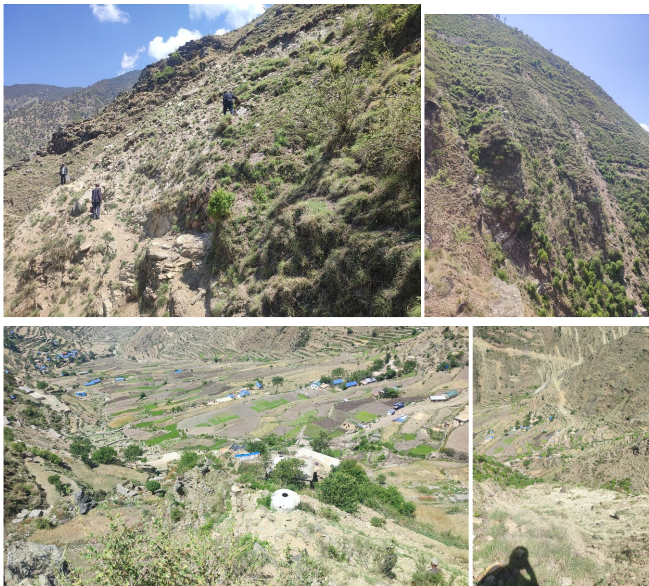
Photograph 92 Landslide Site, Bhita
