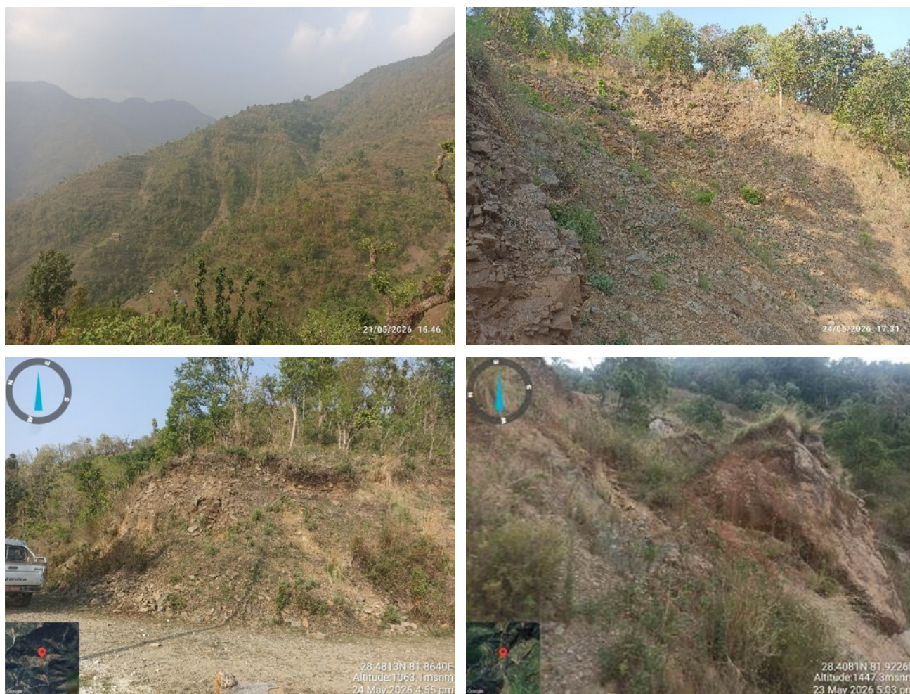
Photograph 88 Landslide Site, Lamidanda
