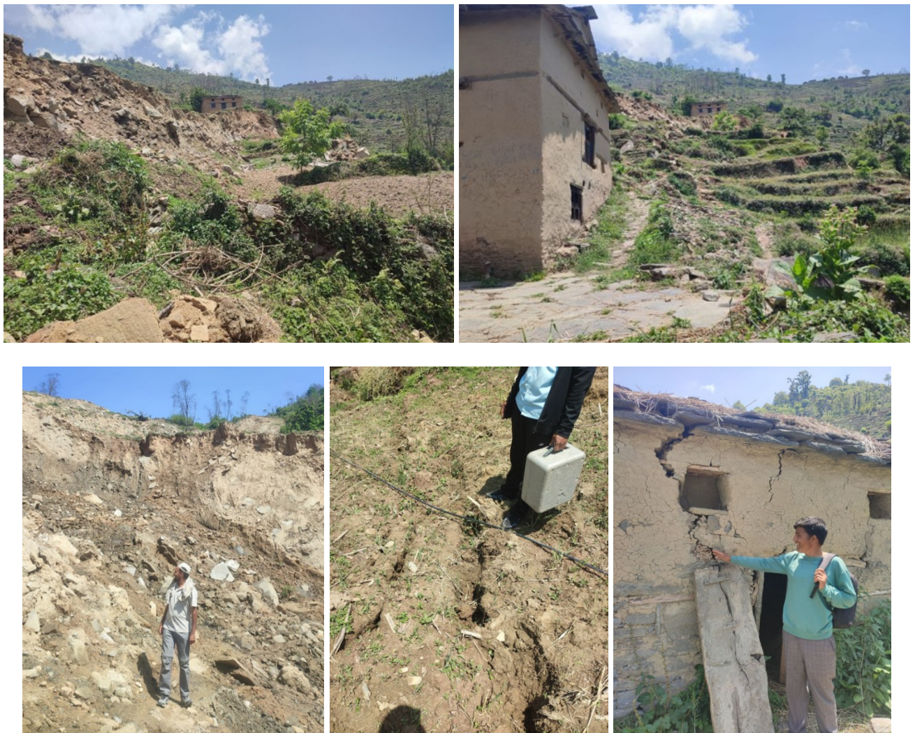
Photograph 95 Landslide Site, Rupsa
